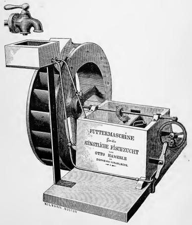
Self-working Machine for feeding Trout.
