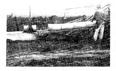
FIGURE 4. CONCRETE PIPELINE INSTALLATION
