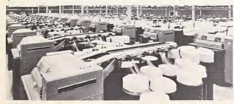
Figure 18 Drawing — The drawing process follows carding except for combed yarns. This process improves the uniformity of the sliver by converging six or eight slivers and passing them through four sets of rolls, each revolving at a different speed, which draws them out without twisting and reduces them to about the same diameter as one of the original strands.
