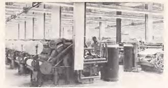
Figure 17 Carding—After the picking process comes carding, which completes the cleaning action, removes short fibers, provides the first step toward bringing the fibers in a parallel order and produces a thin filmy sheet or web which is condensed into a rope-like, but untwisted strand about the size of a broomstick, known as a sliver.
