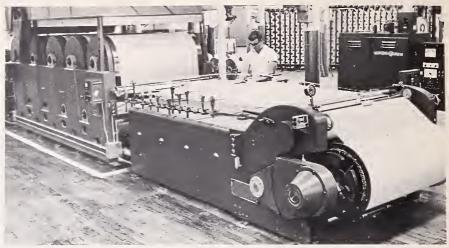
Figure 22 Slashing—After the warping process, which consists of rewinding the yarn onto large warp beams containing several hundred strands, thousands of yards in length, the thread is coated with a thin layer of starch or sizing by a process known as slashing to prevent breaking and chafing of the yarn in the loom.
