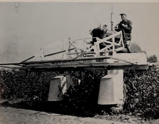
types of topping machines have been built, but the type shown in figure 8 is the most common. It consists of four horizontally revolving blades (one blade to a row) mounted under a frame on the front of a high clearance tractor.
