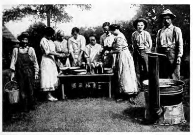
FIG. 55.-Canner made of tubs for outdoor use.
