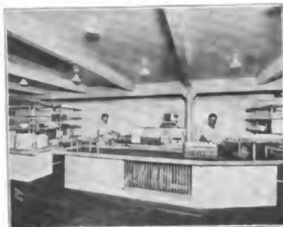
**CHINA WASHING DEPARTMENT**, (Davenport Hotel, Spokane): Blakeslee No. 80 Niagara motor driven machine. Van's new style metal dish tables. Baskets filled and slid to feed end of the machine, passing thru it from right to left and landing on the clean dish assorting table. Tray rack under dish table. Trays are washed in sink in front of the machine (see faucets over tray). Note sanitary enclosure of the dish table.
