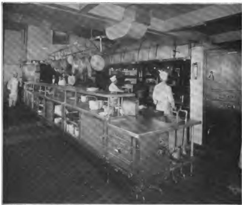
COOKS' TABLE of polished steel in front of range and boilers (Davenport Hotel, Spokane). Special steak warmers are located over the charcoal broilers. A gas salamander is located over the center of range. The hood is specially designed; the exterior of aluminum-coated steel with polished trimmings, and insulated with quarter-inch asbestos board; the main body of hood constructed of No. 14-gage steel.
