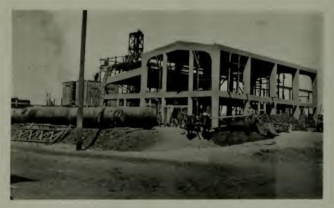
FIG. 6.—CONCRETE FRAME, SULPHUR DIOXIDE BUILDING, AVON, CALIFORNIA Engineering Department, Associated Oil Company
