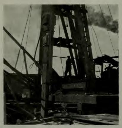
Driving an eighteen-inch octagonal pile 25 feet long and made of Lumnite cement, twenty-six hours after casting. McLain Contracting Company, Baltimore,
