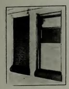
TYPICAL INSTALLATION OF UNDERWRITERS LABELLED FIRE SHUTTERS, PROTECTING WINDOW OPENINGS.
