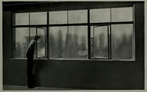
TYPE OF STEEL SASH USED FOR LOFT BUILDINGS
