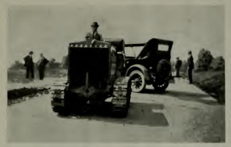
This pavement, made of Atlas Lumnite cement, carried heavy traffic the day after construction. Illustration shows fifteen ton oil distributor and ten ton tractor being driven over pavement twenty-four hours after being laid.
