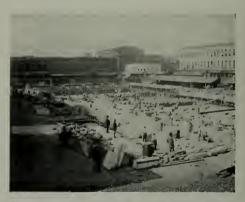
Photo shows start of construction of old Appraisers Building (1874). Note hand concrete mixers, wheelbarrows and foremen wearing stove-pipe hats to distinguish their official station.
