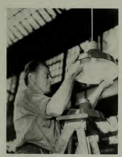
Remavable reflectors make it possible for the maintenance man to remove a dirty reflector and replace it with a cleon one that is carried as an extra.
