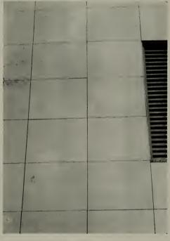
The mortar used in the quarter-inch horizontal and vertical joints (but not elsewhere) for setting and pointing the Ceramic Veneer was mixed as follows:
