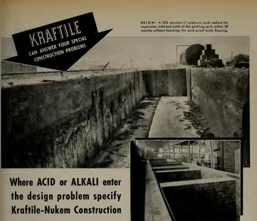
Showing how to construct a tank of Kroftile brick and Nukem jainting compound so as to resist high cancentrations of almost any acid and withstand hard usage year ofter year.
