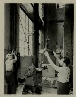
Lowering a luminaire to the floor where it may be cleaned more conveniently is quickly accamplished with the aid of an automatic disconnecting hanger in this high bay area.
