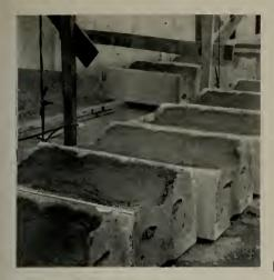
In above photograph, note that the wash surface at vertical joints is cut out to provide grout holes which enable the vertical joints to be grouted solid, covering the anchors with mortar. The water-tight vertical joints are finished with a covering of Ceramic Veneer filler pieces.
