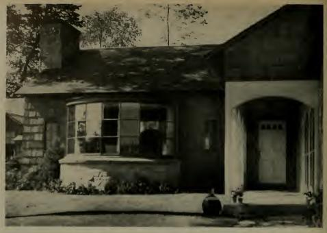
The large squares af "Thermapane" abviate any need for storm sash; they keep heat out in summer and retain it in cold weather. Roof is contilevered to ease laad on sash
