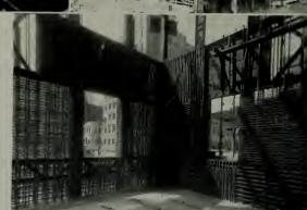
floor acting as a horizontal girder, was designed to distribute the seismic loads to these walls and braced bays in proportion to their relative rigidities.
