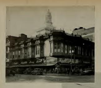
Modernization of the Delger Building called for the removal of bay windows, unadorned roof line and new exteriar without making alterations of the structural elements.
