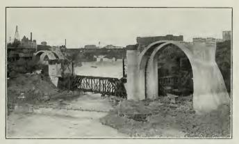
Fig. 1 View Showing Spokane Arch With Steel Trusses in Place to Receive 281-Foot Timber Center
