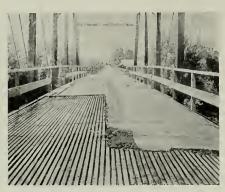
The Timber is Protected from the Rains and will Not Decay. It lessens the impact of the moving load on the structure.
