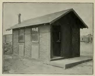
Small Building Erected to Show the Possibilities of Reinforced (Panel) Brick Wark
