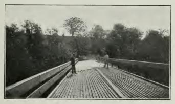
Fig. 2, Showing Timbers Placed Lengthwise of the Bridge, and Concrete Wearing Surface on Deck Span
