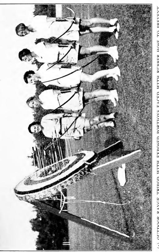
(5) OUTDOOR RANGE TRIPOD WITH EXPOSED PORTIONS FACED WITH RUBBER HOSE TO PREVENT ARROW BREAKAGE OR RICOCHETS
